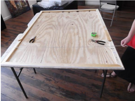
Figure 13. Wire is run through the left D-ring and both ends are cut long on the right
