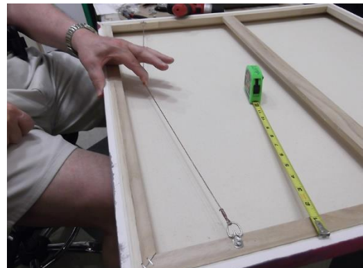
Figure 12. Checking the final wire tightness
