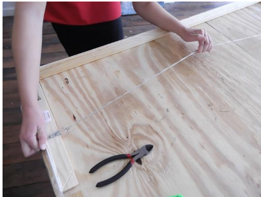
Figure 21. Stretching the twisted wires
